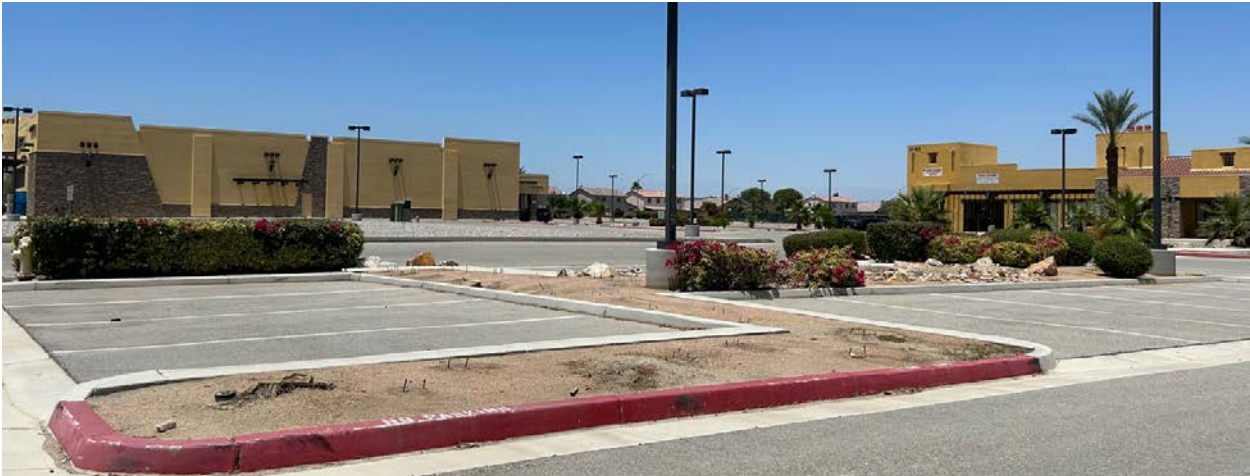
2023 (reverse angle of Internal Landscape Area with missing trees and shrubs)
