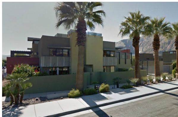
Three-story modern townhouses with tuck-under parking.
