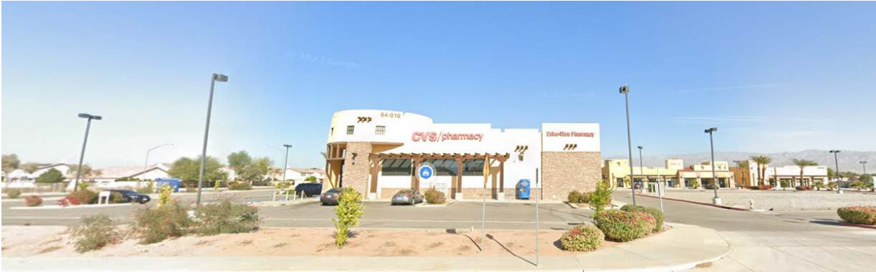
2022 (Avenue 50 Frontage – Missing Trees and Shrubs)
