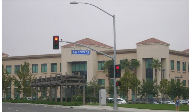
Typical two-story office building.
